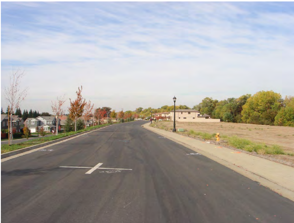
Looking eastward down Rivercrest Drive at The Rivers EIP site. Note vegetation to the right on the waterside, homes on top of the levee crown (Rivercrest Drive), and homes to the left at the landside toe.
