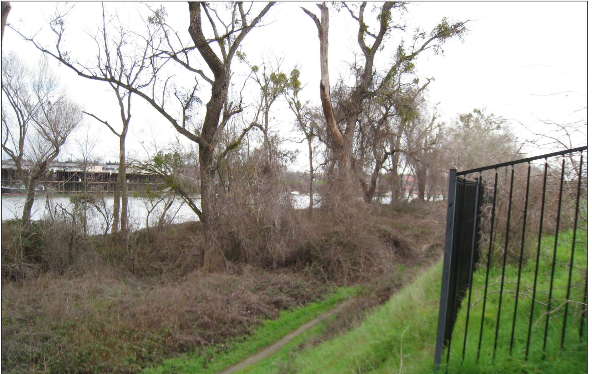
Looking northeast atop the levee crown. Note the fence delineating the property line of a home located on the levee crown to the right of the photo and the riparian vegetation lining the levee in the foreground.
