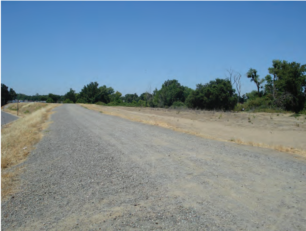
Looking west on the levee crown. Note DWR maintenance yard on horizon at left. Note Riverbank Road at extreme left and mature vegetation at right and on the horizon.
