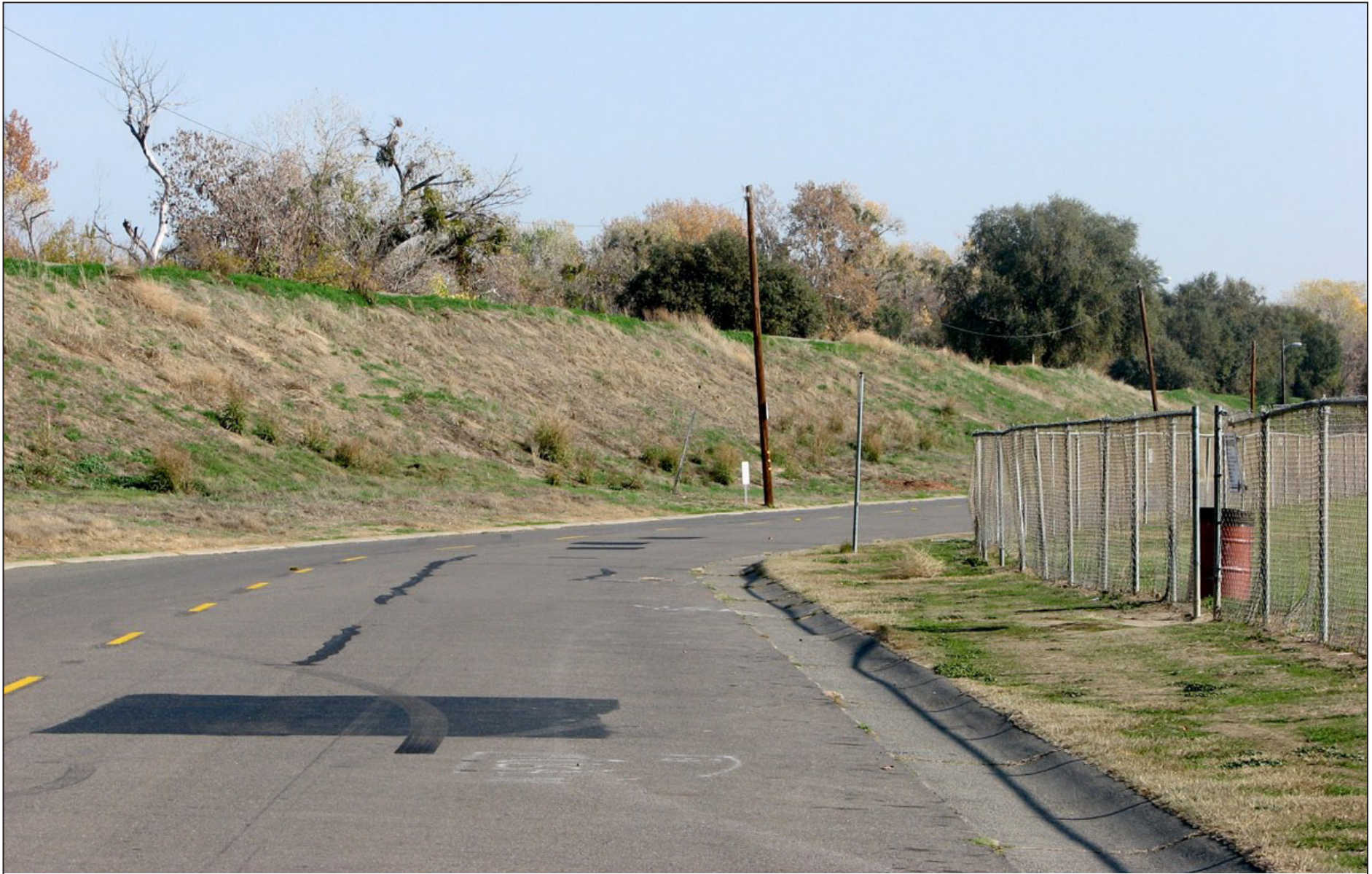
Looking east across Riverbank Road. Note the levee embankment across the middle of the photo with mature riparian trees visible on the waterside. This photo depicts a section of the levee with an open space element.
